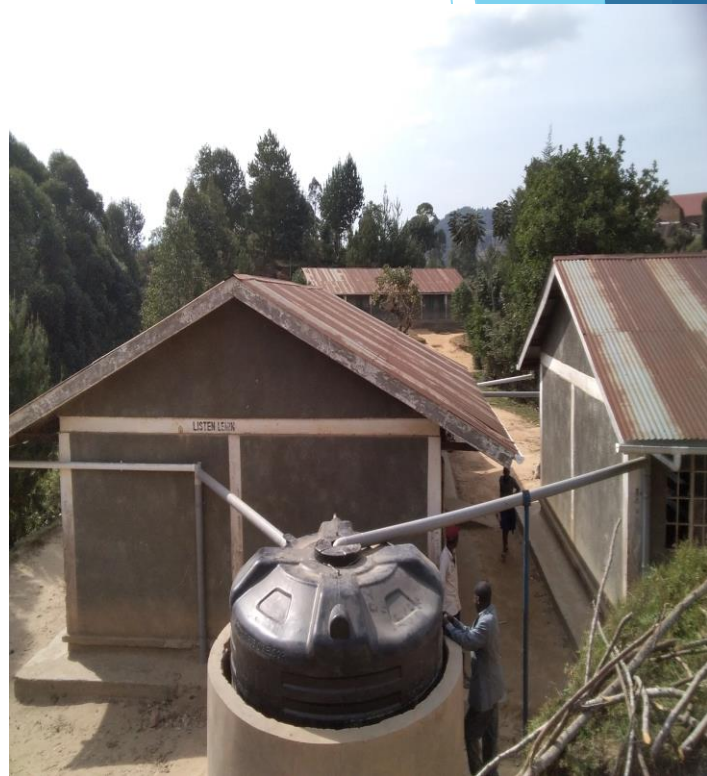
Constructed water harvesting tank at Nombe primary school in Bwindi
